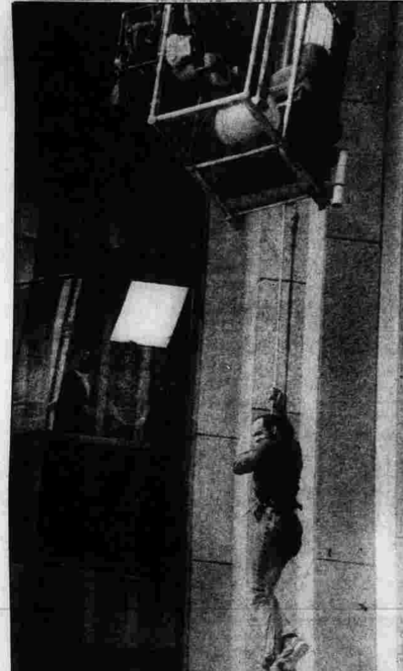
CLOSE CALL — Window washer Charles Cano dangles from a safety rope after high winds up scaffolding he was working on at the Pittsburgh National Bank building in downtown Pittsburgh Thursday afternoon. Two window washers were rescued after dangling from safety ropes and after being taken to Mercy Hospital it was determined neither was seriously injured.
